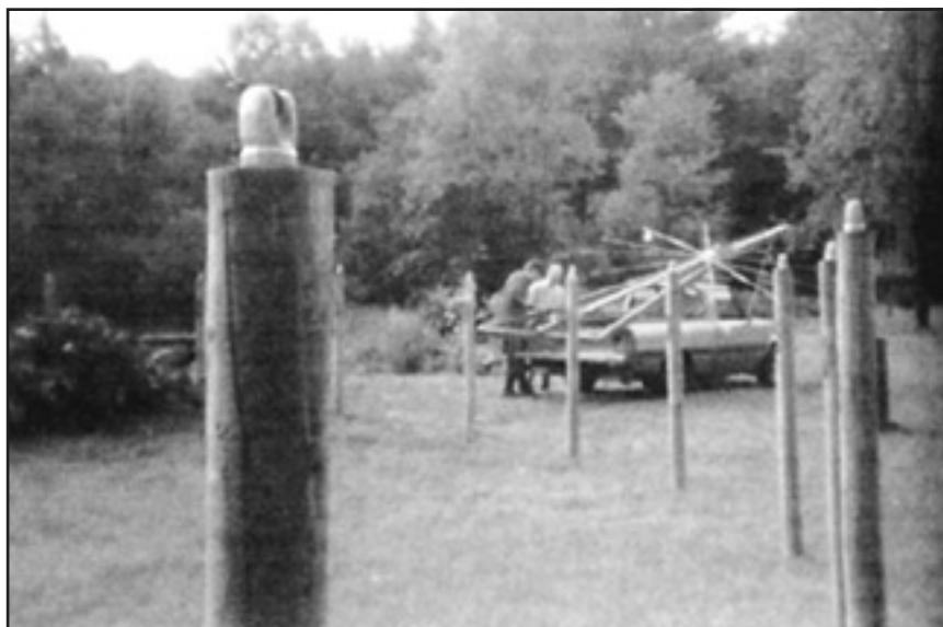
Fig 57 —Photo showing some of the fence posts used to hold individual cone wires to keep them off the ground and out of harm's way. The truck in the background is carting away the A-frame discone for installation at KA8UNO's QTH.
